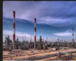
Saudi Aramco shell refinery co.
